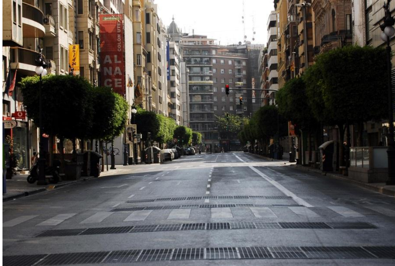
Figure 6: Image with the section type of the inner ring road (Colon Street).
