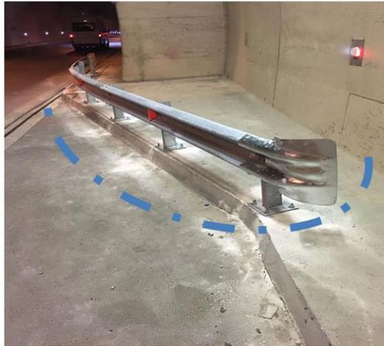
*Installation of guardrail in front of perpendicular wall of lay-by in Krrabe tunnel (source: Hasani A., Albanian Roads Authority)*
