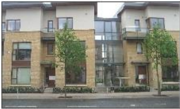
Close Proximity of Buildings
