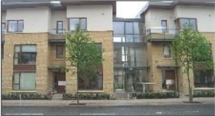
Close Proximity of Buildings
